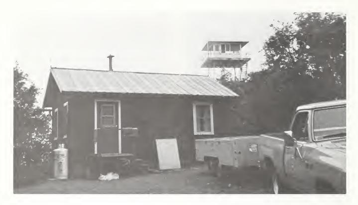
Figure 81. Rose Peak lookout and cabin on the Apache-Sitgreaves National Forests. The lookout is an Aermotor MC-24 constructed in 1929 and then altered in 1981.
